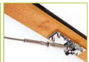
STAINLESS STEEL TIRE WIRES OFFER A MODERN ALTERNATIVE TO TRADITIONAL TIE BARS
